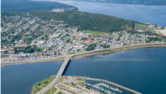
View of the bridge arriving to Gaspe
